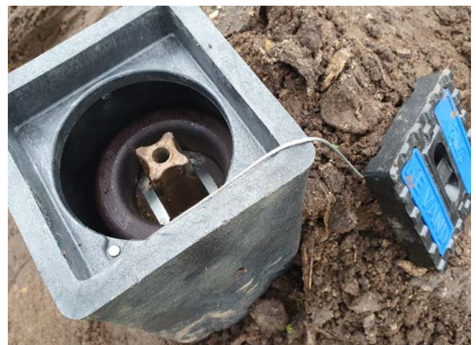
The VIDI Positioner installed in a plastic surface box.
